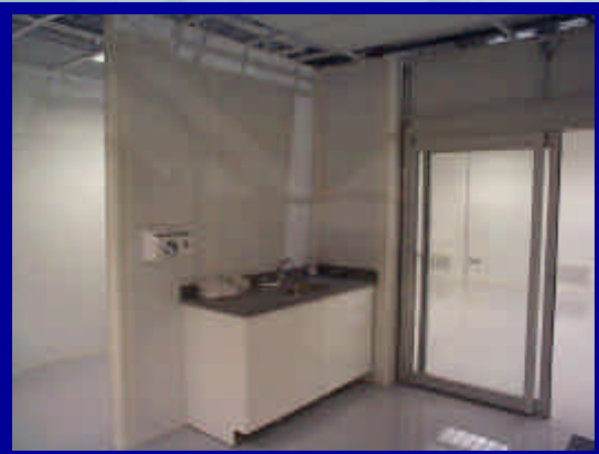
Sink & Hand Dryer Double Electric Door
